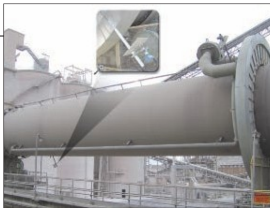
FIGURE 4. This cement kiln rotates almost twice per minute and operates at temperatures up to 2,800°F — a case in point where wireless instrumentation excels over wires
